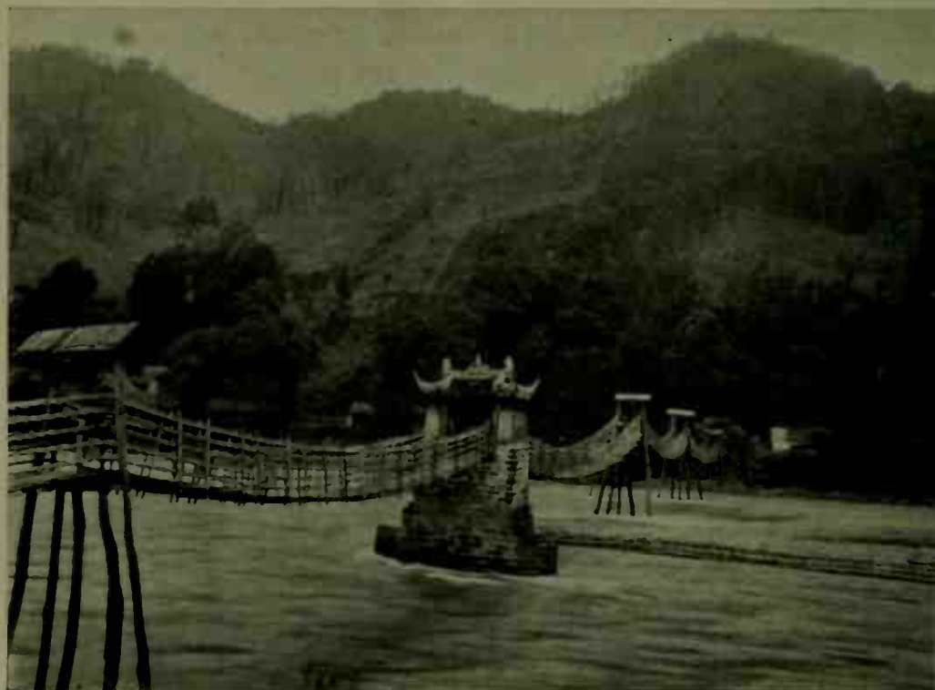
The great suspension-bridge of bamboo cables across the river at Kwanhsien is ethnologically the dividing-line between China and Tibet, though politically China stretches many miles farther westward
